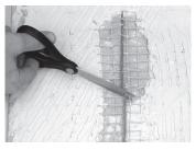
Step 3.1. Cut out the damaged wire location, creating two ends or leads. If the cable being repaired is not the jacketed heating cable, skip to Step 3.6.
