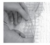
Step 3.9. Pull the braid straight out to make it into a pigtail.
