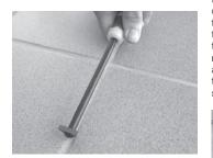
Step 2.1. If not done so already, carefully remove the tile/stone/marble floor covering over the damaged cable area. Removal of the grout around the affected tile(s) must be done with a blunt instrument such as a hand-held grout-removal tool. **DO NOT USE A KNIFE!** Gently break out the tile with a small hammer, removing the fragments as the tile is broken up.
