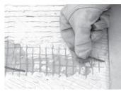
Step 4.5. Use a glove or other protective cloth to pull off the loosened jacket slug. Do not touch the hot jacket slug with bare fingers. The slug will be very hot and will burn!
