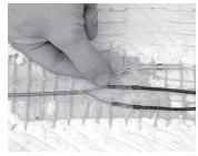
Step 4.21. At the other end of the ground jumper wire, slide a ground solder tube over the wire. REPEAT Step 4.20 to complete this connection. Be sure to avoid reheating or scorching the heating wires or splices, using a heat shield again if needed.
